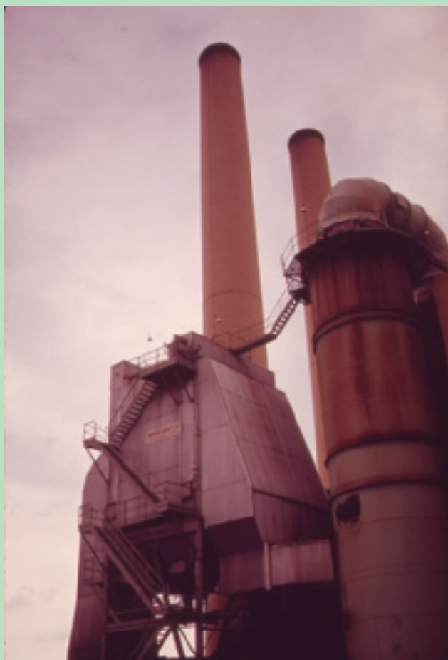
This is an industrial-size electrostatic precipitator. Residential ESPs are often marketed as "air purifiers."
